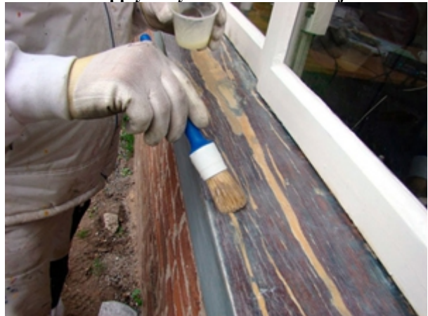
Apply a second layer of Renofix Oranje (wet in wet)
