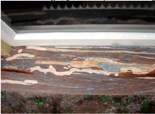
Repair larger cracks.
